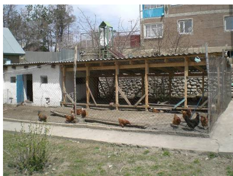
Chicken house showing new roofed area providing protection from the elements
